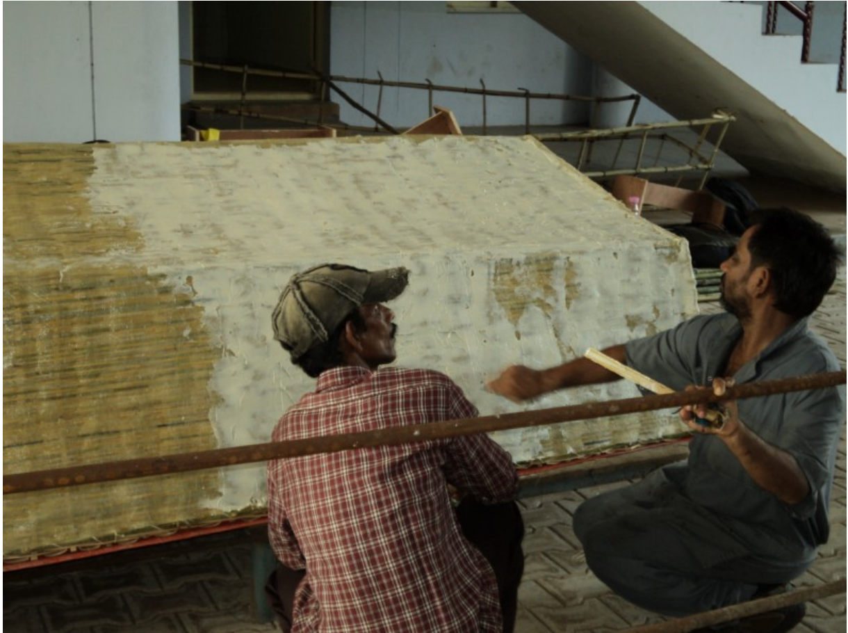
SPECIAL HIGH-STRENGTH PUTTY COMPOSITE APPLICATION
