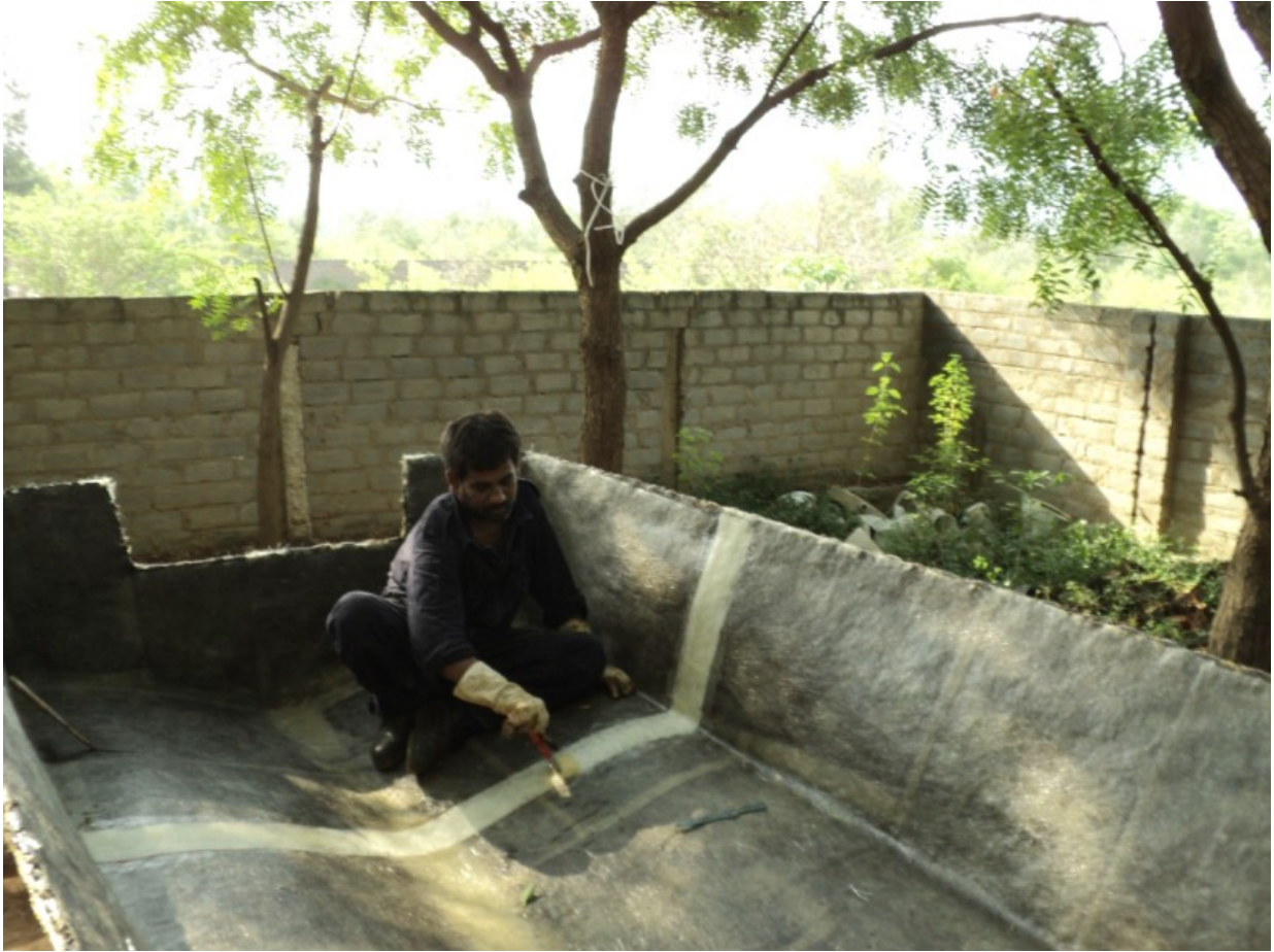
INNER LAYERS BEING STRENGTHENED WITH GLASS-FIBER SYSTEM
