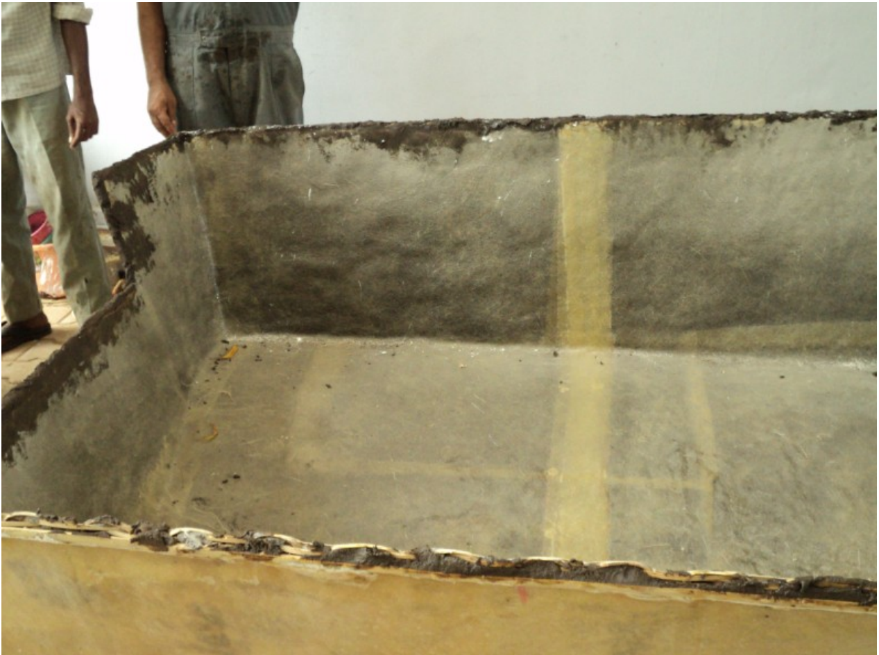
INNER LAYERS BEING STRENGTHENED WITH GLASS-FIBER SYSTEM
